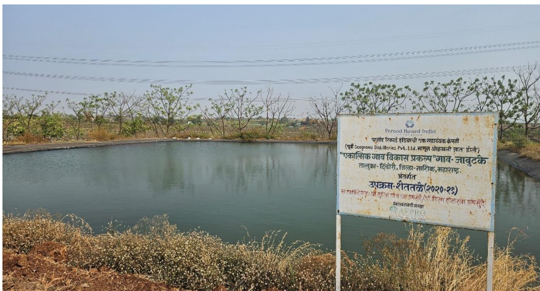
Figure 12: A poly pond established under the programme in Jambutake village
